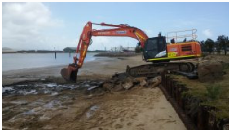
Concrete being removed
