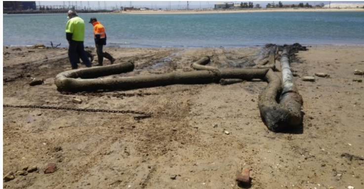
Industrial waste pipe about to be removed
