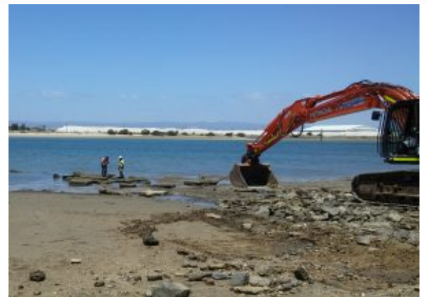
Sheet metal being dragged off shoreline
