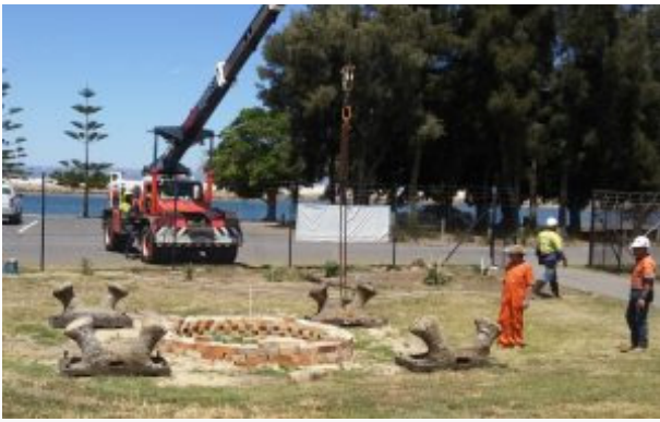
Shane Walter (PASC) Checking Bollards in place
