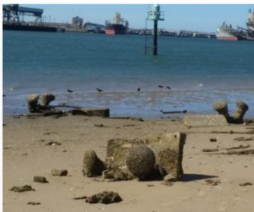
Mooring Bollards on shoreline
