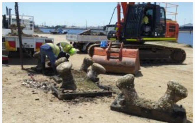
Cleaning the Bollards' bases
