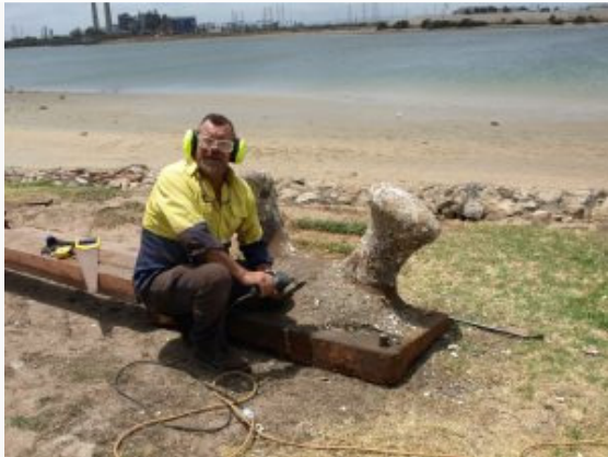
Lyndon Zimmermann Preparing Bollards at GST Dolphin
