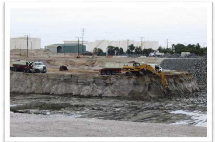
Excavation of the new Marina at the Acid Plant Site
